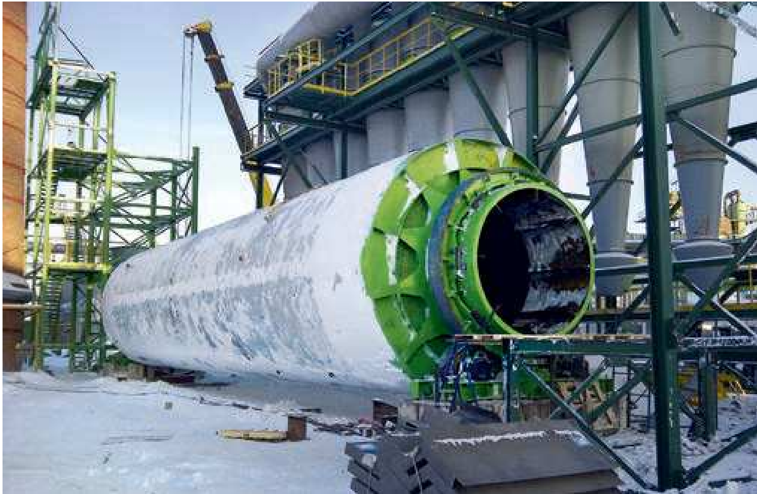
Installation works on the Büttner drum dryer
